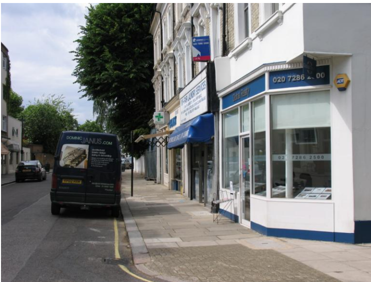
The eastern side of the local centre, containing important services such as the pharmacy.
