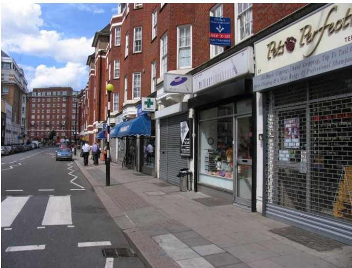
The southern end of the core frontage, showing closed and vacant shop units in the local centre.
