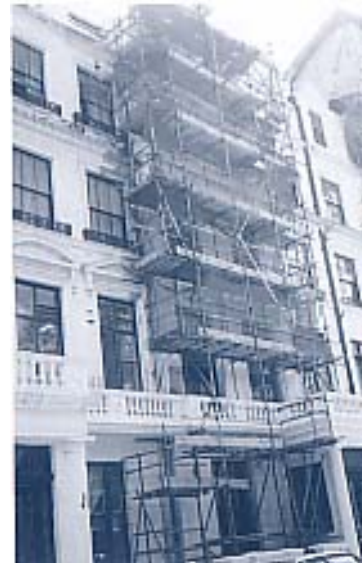
Fig. 5: Left: Example of scaffold covered with impervious plastic sheets which may, in some cases, act as 'sails' and pull down unsecured parts of a wall.
