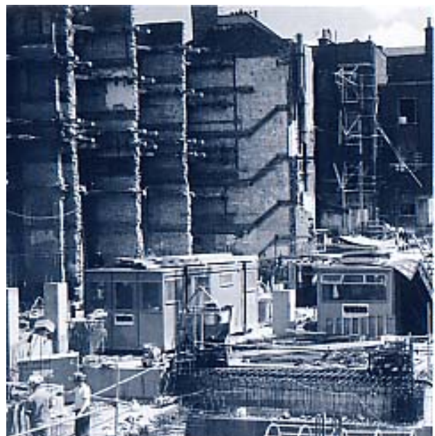
Fig. 12: Radical alterations to historic buildings (if they are acceptable in other respects) may involve retention of the facade with total demolition of the structure behind. In such cases, the retained facade is vulnerable to collapse, unless it is adequately held up by temporary supports.
