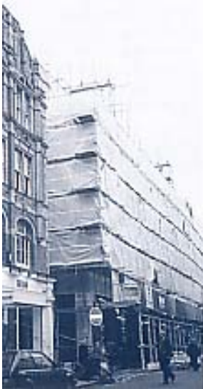
Fig. 5: Left: Example of scaffold covered with impervious plastic sheets which may, in some cases, act as 'sails' and pull down unsecured parts of a wall.
