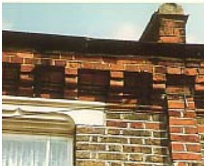
***The projecting brickwork or corbelling below the eaves is very exposed to the elements. As a result the soft red bricks can become badly eroded.***
