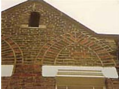
***In this photograph the poorly applied pointing has overwhelmed the subtle textures of the brickwork. Compare with the more appropriate pointing between the window arches.***
