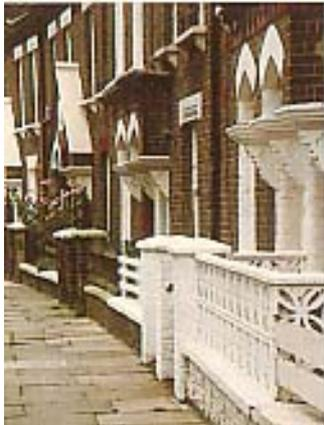
***Modern types of front garden walls can spoil the uniformity of the terrace. When replacing or repairing use the appropriate cast iron railing and dwarf wall.***
