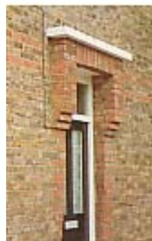
***In this photograph the porch has been rebuilt in a simplified form with all elements of the original design omitted. Alterations of this type will be resisted through the Article 4 Direction.***
