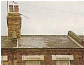
***Care should be taken to ensure that the replacement slates match the original colour.***
