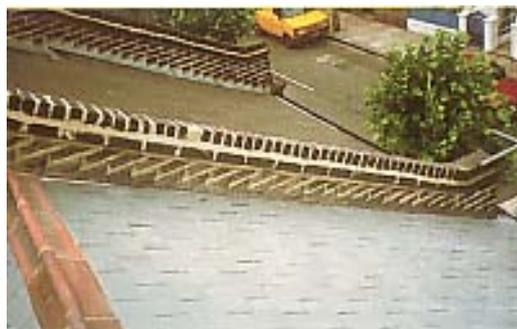
***Lead flashing at the party wall should be stepped into the brickwork but, unlike in this example, care should be taken with the mortar mix to match the colour and texture of the original.***
