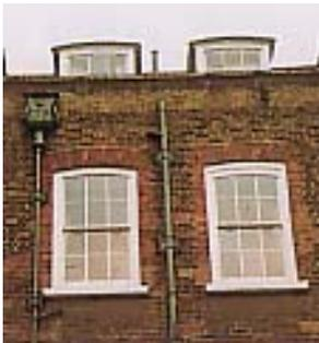
The roof of the dormer should normally be flat. However, in some cases it may be acceptable to use a shallow curved roof to reflect the design of window openings on the façade.
