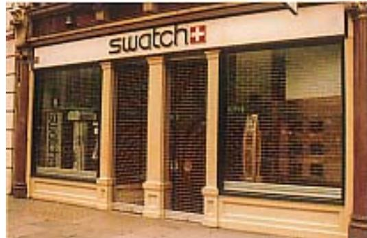
***External lattice and Brick Bond grilles, set between the existing architectural details of a shopfront.***
