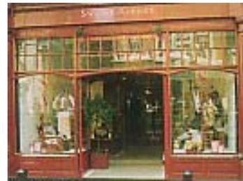
The use of laminated glass in shopfront windows and doors should be the first option as this has the least impact on the appearance of the shopfront and would not normally require permission (unless the size or position of the glazing frame is altered). However, in cases where historic glass (Crown Glass) survives in the shopfront window of a listed building, consent would be required for its replacement with modern glass.
